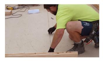
Refer to the Lockwood production plans and mark out, tie rods and electrical cable locations on the finished subfloor. Check your measurements carefully against the Lockwood production plan dimensions.
