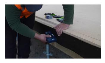
Install PVC base flashing by clipping it onto the Seating Profiles. Press firmly on the joists and fix with nails. The corners need to be mitred and all joins sealed with silicon.
