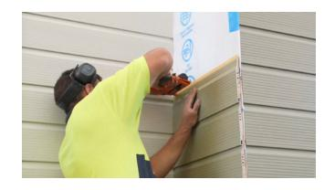
Seal exterior corners using a suitable flashing tape before installing Corner Profiles
