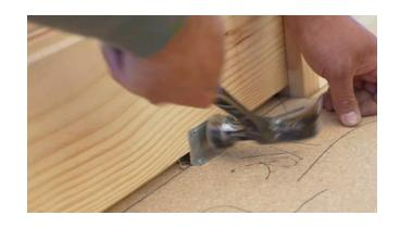
Install PVC wedges in the exterior board scallop wherever the board meets a window, door, wall joint or corner.
