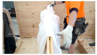
For a short-term solution on partially built walls, use the timber dunnage from the Lockwood delivery trimmed to length and nailed to the top tongue.
