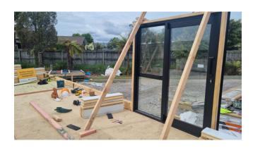
Lift sliding doors into place. The door rollers will be lifted as high as possible to allow for easy installation. Rollers will need to be adjusted for the sliding doors to operate and rechecked and adjusted at the completion of the build.
