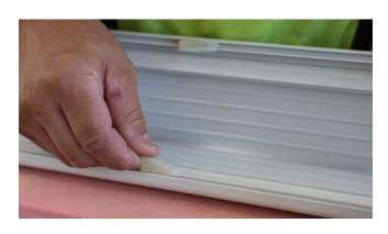
Fit an aluminium L Profile into internal corners sealing it in place. Seal meter box with RTV silicone sealant and install W repair profiles
