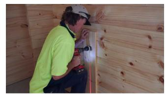
Cables are installed down through the power holes in the sarking and pulled through socket and switch holes using cable pullers.
