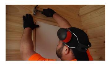
Use 44 cappings to cover the end grain of the internal walls. Cut them to the required length and nail them in place.
