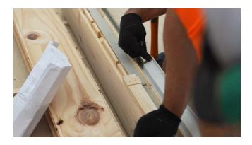
Fit wind seal to the underside of the head flashing allowing 50mm from either end. Then install the lintel boards above the windows, ensuring they are square and plumb once complete.
