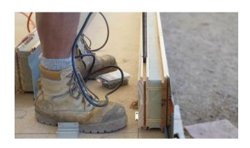
Mark out the position of full height stiffener and beam posts and install two multi-grips or J9 brackets for fixing to the side of the post
