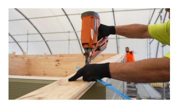
Fix the sarking boards at the top structural support – either a ridge beam or a wall. Then fix at the bottom structural support – usually the top of an external board.
