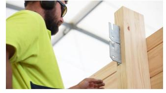
Remove the beam bullnose so the beam will sit flat against the post.
