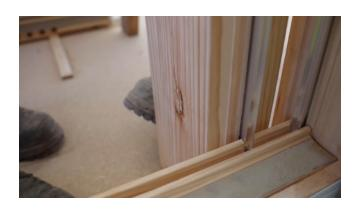
Install 'X' Profiles as you work your way up the wall. Leave a 200mm gap between the first and second profile using a temporary nail to hold the profile in place. This makes it much easier to install the interior boards.
