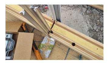
At two boards high, fit full height stiffener and beam posts into place using an 'X' Profile. Fix with multi-grips.
