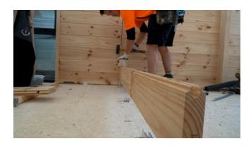
On timber subfloors, with the bottom boards in place, drill tie rod holes through the floor.
