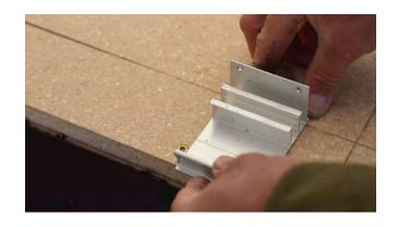
Fix interior seating profiles with two nails as preparation for first interior board installation. Place at 900mm centres and either side of any openings, avoiding tie rods.
