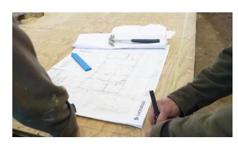
When setting out, dimension everything from one exterior side and one exterior end of the floor as a fixed measuring point.
