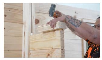
At three boards high, knock the 'X' Profile down to allow for the next three boards to be installed.
