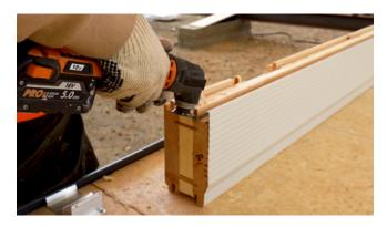
Install the first boards over the Seating Profiles, referencing the Lockwood Production Floor plan. Careful attention to the outline and position of first boards will ensure a smooth build.
