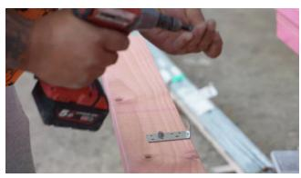
Use the consent and engineering plans to identify dummy rafter placement and fixings. Install at the specified centres.
