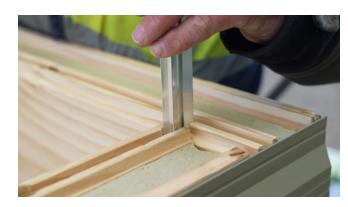
When all exterior first boards are installed, fit full height 'B' Profiles where an exterior wall uses butt-joined boards. Install PVC wedges as you install the 'B' Exterior profiles.
