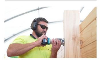
When positioning brackets, check the beam will be level once fitted
