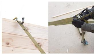
Fix a temporary cap to door openings and wall ends to keep them plumb.
