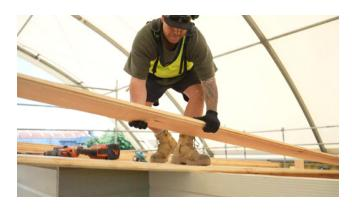
As you fit the sarking, watch for upcoming tie rod and electrical holes. Measure the position of the hole from the tongue of the previous board and note this on the board that will cover the hole.
