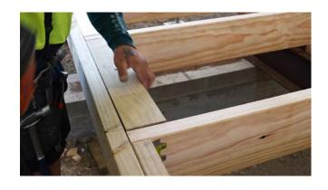
Fix Tie Rod Nogs in place with nails, screws and four multigrips.
