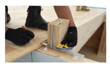
Provide continuous temporary support under any sarking spanning 2.5m or more. Keep this in place until the roof is fixed.
