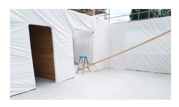
If rain is expected, use the supplied rolls of white plastic to cover up. Drape over walls and secure to the floor.
