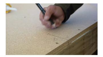
Check recess sill depth and widths on the Lockwood Production Subfloor Plan. Cut recesses out of the flooring to allow for the full height/ floor set door and window joinery.
