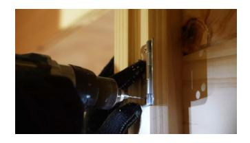
Hammer home jambs and head after the doors are hung. The fit of the doors can be improved by the way the frames are hammered home.
