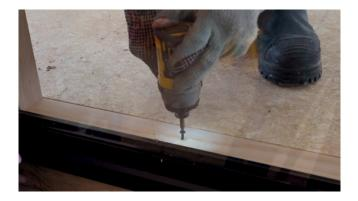
Ensure the frames are square and plumb, and securely brace full height joinery to the floor.
