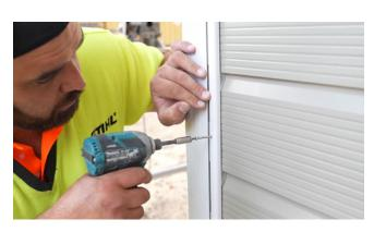
Timber boxed corners come in two pieces, Fix the smaller edge on the front face of the exterior wall, nailing every four boards.
