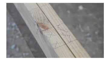
Identify tie rod nog and full height sill nog locations on the Lockwood Production Subfloor Plans.
