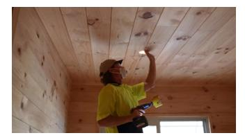
Every wiring hole should be patched with squares of sarking overlay, extending a minimum of 100mm from the holes and securely sealed with tape.
