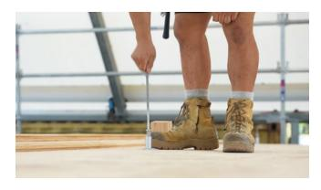
For timber subfloors, fit a 50x50mm washer and nut at the base, the nut should be screwed on only slightly past the bottom of the thread.
