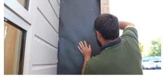
Install base clips at the bottom of the wall to be over lined.
