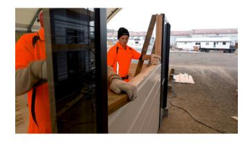
Install PVC wedges in the exterior wall scallops wherever the board meets a window, door wall joint, or corner before placing the next board.
