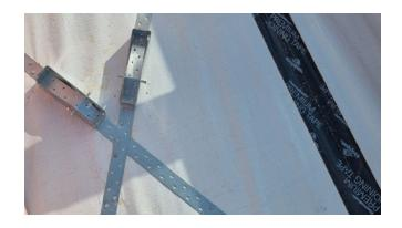
Screw fix every second sarking board to the outer edge of the wall. This straightens the boards and makes it easier to fit rebated fascia.
