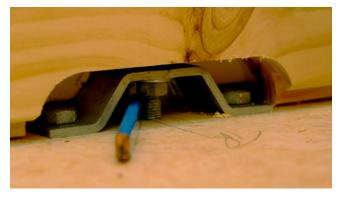
Tension the tie rods as required or to help close gaps due to board growth. It's important not to over-tighten. Use hand tools, not a torque wrench or other power tools
