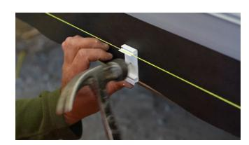
Fit the flashing baseboard by clipping on to the clips. You may need additional clips at joins.
