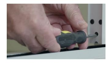
Install 'X' Profiles on each side of the joinery frames joining them to the bottom boards.
