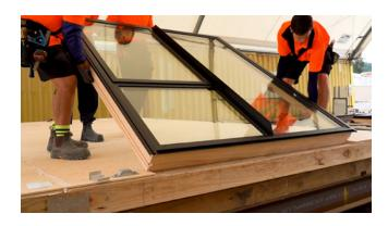
Use 50mm screws at 500 centres to fix the sill down to the recessed sill nogs, or into the double joist at gable ends.
