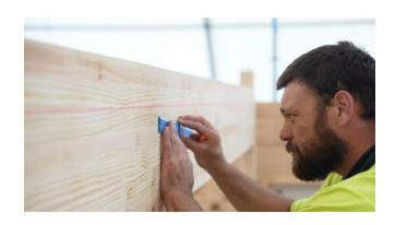
The main ridge beam should be fitted first, and gable walls should be checked for plumb before installing the other beams. Use string lines to line up and level beams.
