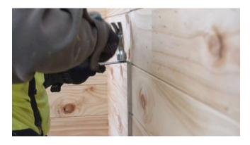
Ensure V grooves are lined up as you go and check wall heights as you build.
