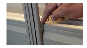
Check the Tie Rod and electrical holes match up with the marks previously made on the subfloor. Remeasure, check the Lockwood Production Floor Plan and amend if required.
