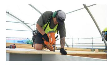
Bring the next board into place. Skew nail the top of the previous board again before fitting the next one. This tightens the sarking as you go.
