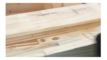
Measure out and drill tie rod and power holes as you go. Tap a nail in next to the hole to help identify their locations once the sarking overlay paper is installed.
