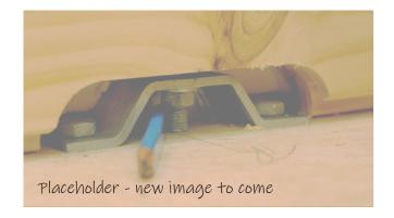
Prepare 'X' Profiles for easy installation. Some builders like to tap the ends of the X Profiles to make fitting easier.
