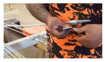
For sea spray zones, a tie rod pack will be supplied with a stainless steel nut, washer extension and coupling. Attach these to the bottom of each rod before installing in tie rod holes.
