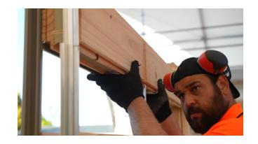
Install windows as you build the exterior walls making sure they are tightly in place. Build the wall up to the top of the window adding 'X' Profiles and PVC wedges as you go.
