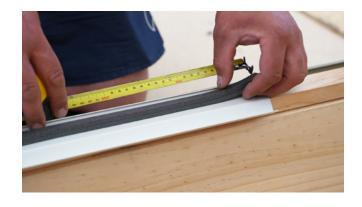
Check the height of the V between the 12th and 13th boards; this should be 2074mm from the floor and no more than 2077mm. Any more would indicate board growth.
