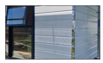
Trim corner Profiles to length and install PVC Wedges before fitting. On timber boxed corners, the PVC wedges fit into the outer weather groove furthest from the corner.
