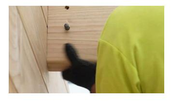
Mark beam checkouts on wallboards and intersecting beams. Before cutting, double check measurements against the Lockwood factory plans.
