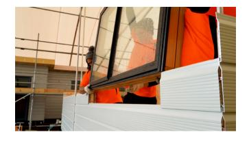
Fit the head packer and head flashing to the lintel board. Head flashings are cut to length and should extend equally on each side of the headpacker. Fix the head flashing to the tongue of the lintel board to avoid head flashing creep.
