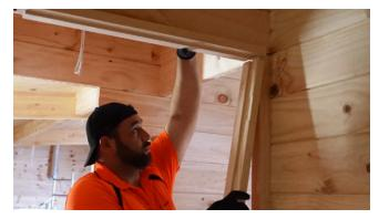
Install hinges and hang doors. The door leaf should have a gap of around 1.5mm on the hinged side and 3-4mm on the latch side. Ensure the gaps are even all the way up the door.
