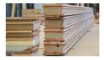
Stack the boards with the labelled side visible at one end and check the power and tie rod holes line up.
