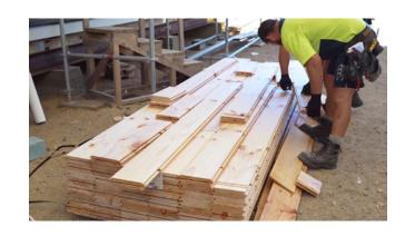
Each wall is designated with a letter shown on the Lockwood Production Floor and Wall Plans. Each board is labelled with the wall letter and a number to denote its placement.
