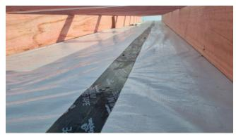
Fix the sarking straps and tension using the kit provided. Sarking straps help tighten the structure and are required for all spans greater than 2.5m.
