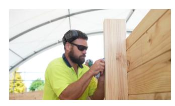
Check beam labels against the Lockwood factory drawings to identify locations.
