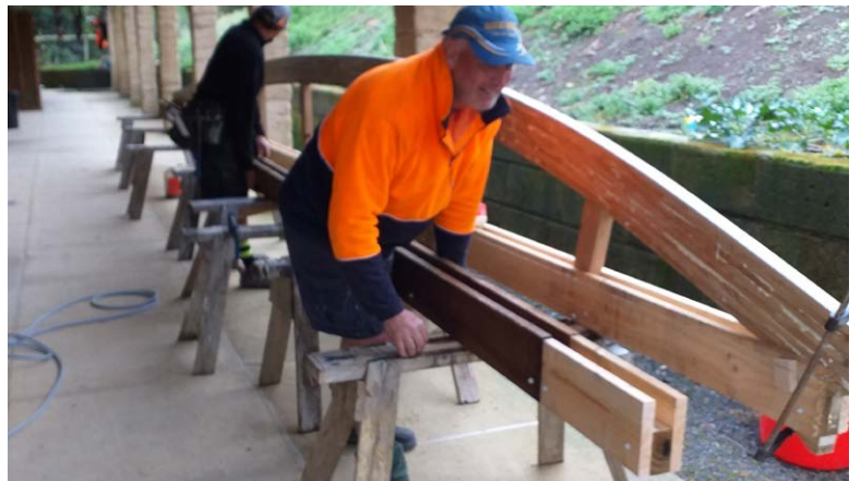
^The beams were made in stages, using moulds and clamps
