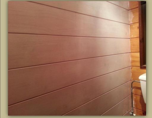
One full coat of Timbakote applied to the left hand side of the toilet wall
