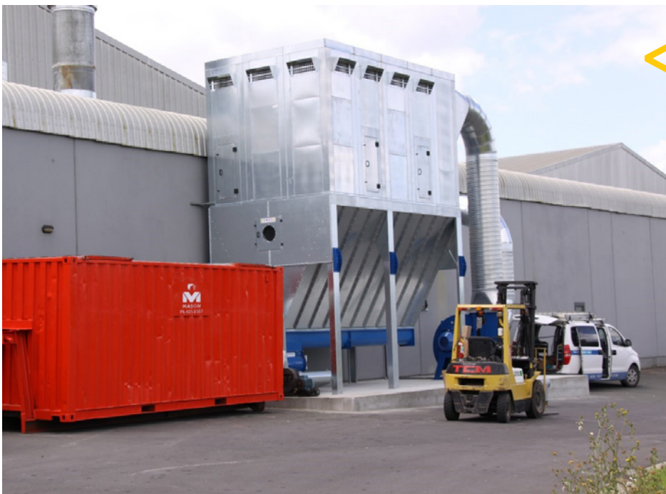
Similar unit to the two extraction units to be each installed for Joinery and Precut.
