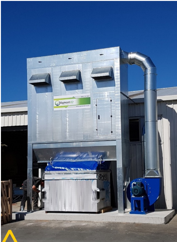
Similar unit to the two extraction units to be each installed for Joinery and Precut.
