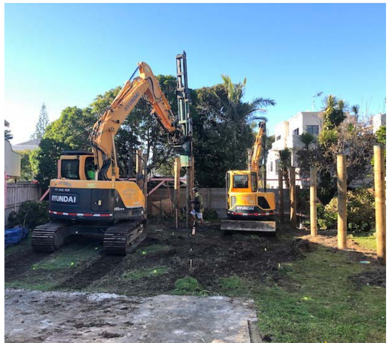
The tight urban site was a challenging space to build in.
