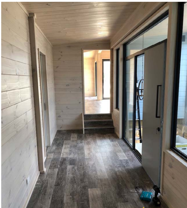
Split levels allowed for car parking underneath the home
